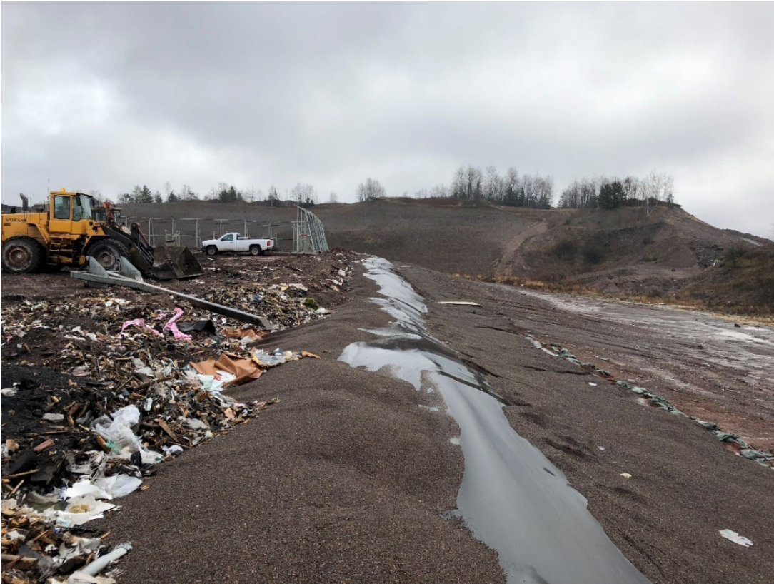
Photo 33: Location 12 – Looking East, Cell 7A Southern Rain Flap
