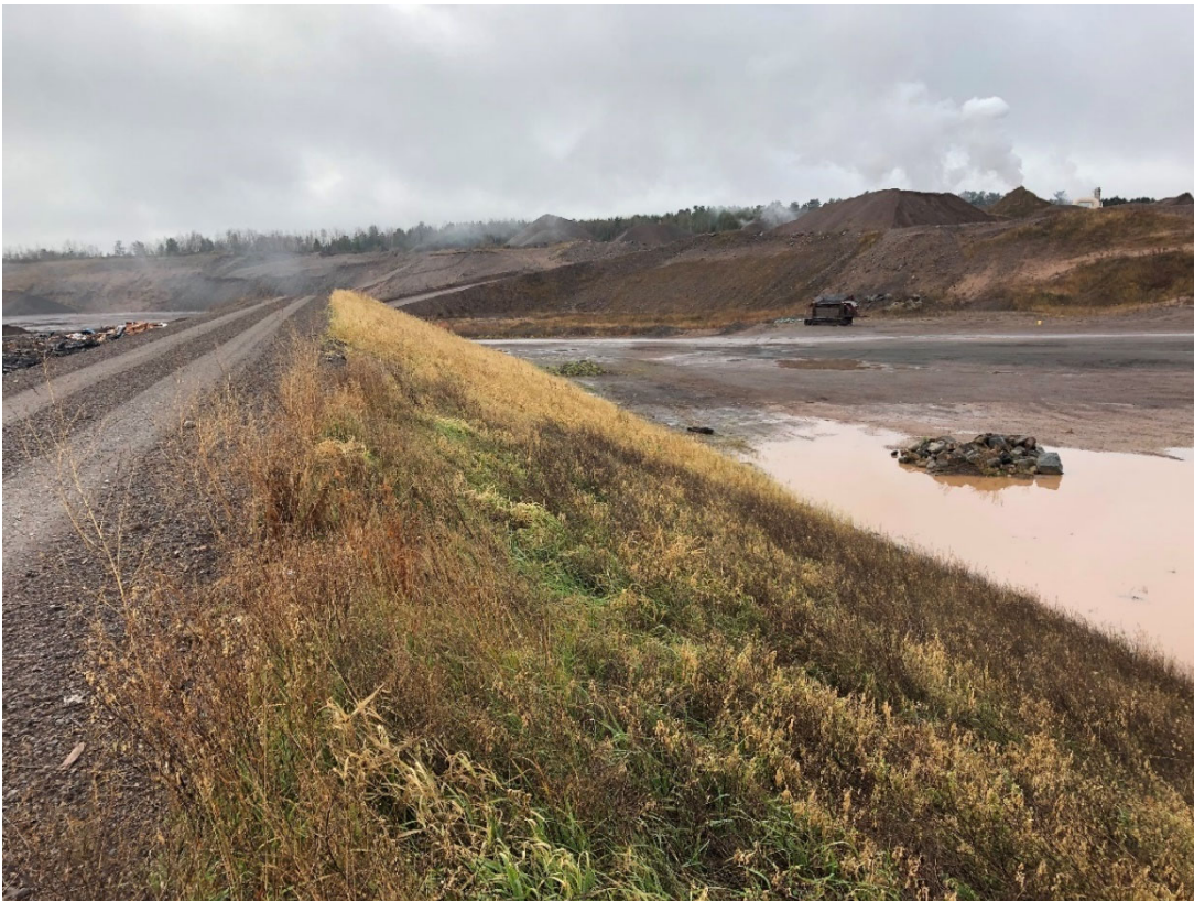
Photo 16: Location 8 – Looking South, Phase 6 Western LF Berm
