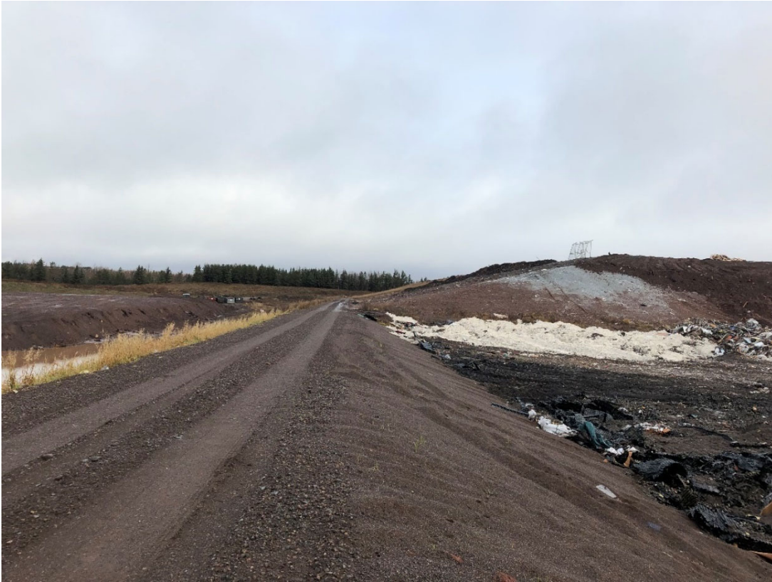
Photo 29: Location 11 – Looking North, Phase 6 Interior (Future Waste Slope)
