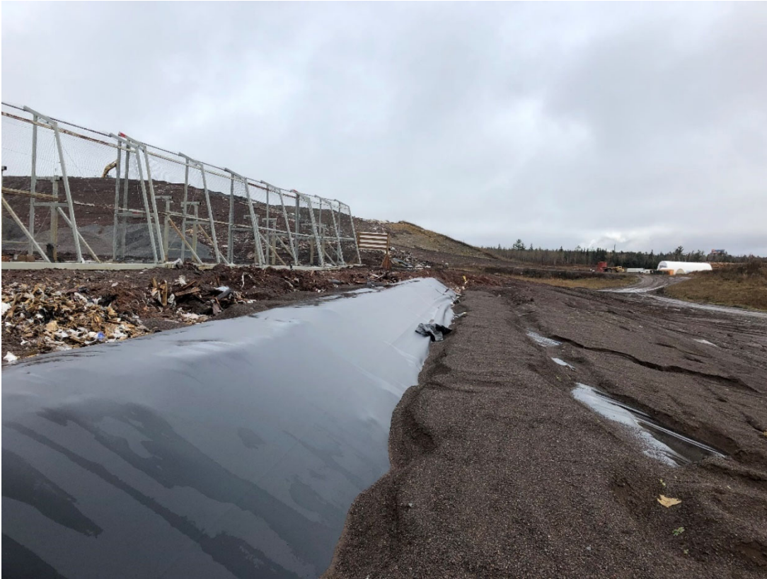
Photo 35: Location 13 – Looking North, Cell 7 Eastern Berm
