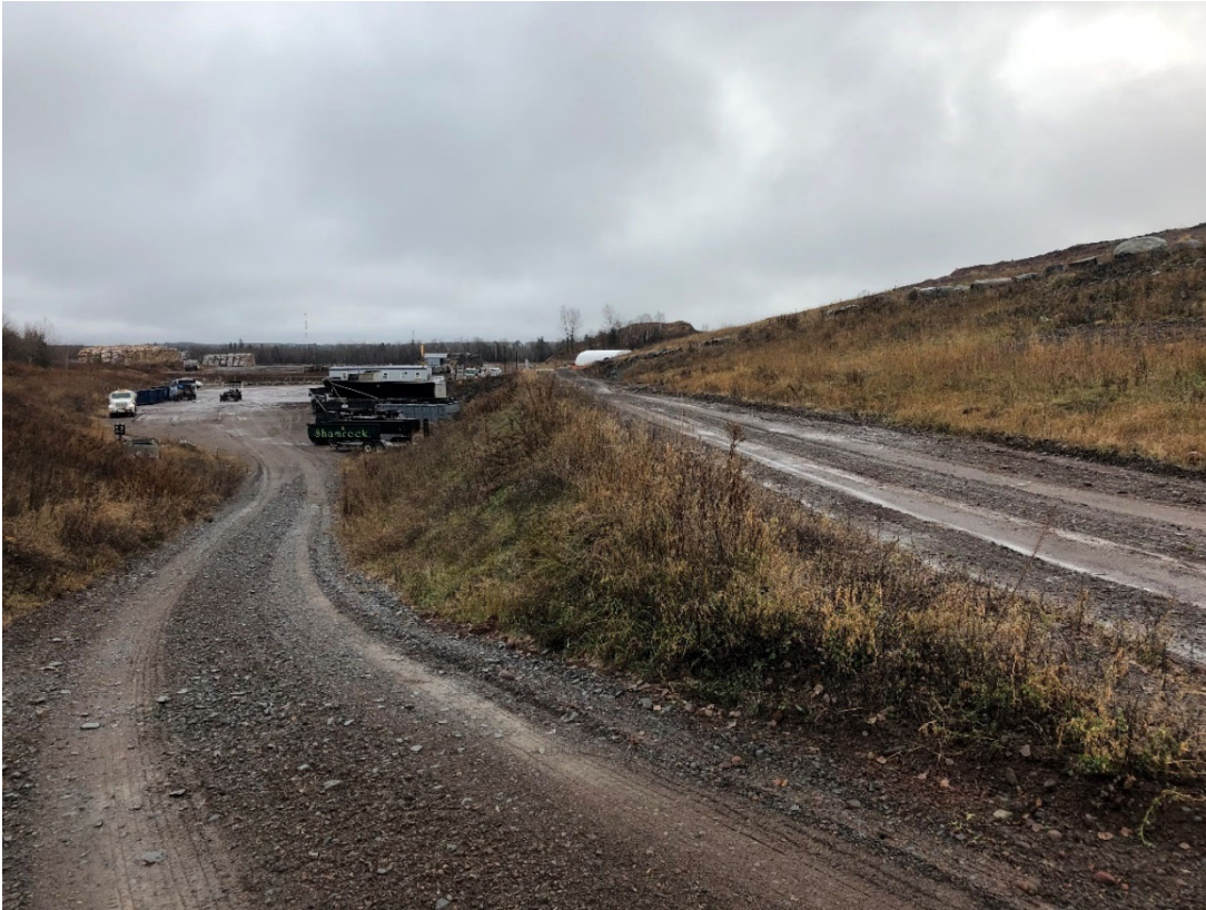
Photo 27: Location 10 – Looking East, Phase 2 Road & Berm
