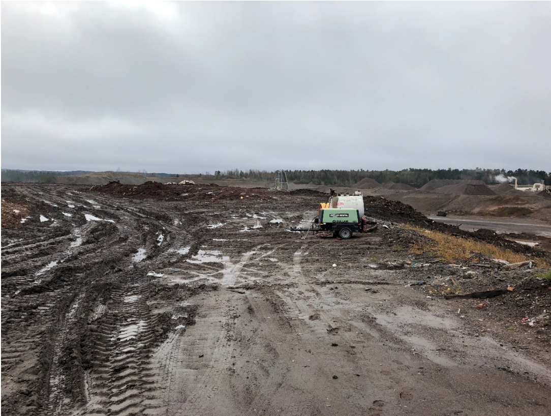
Photo 1: Location 1 – Looking South, Phase 2/3 Upper Lifts
