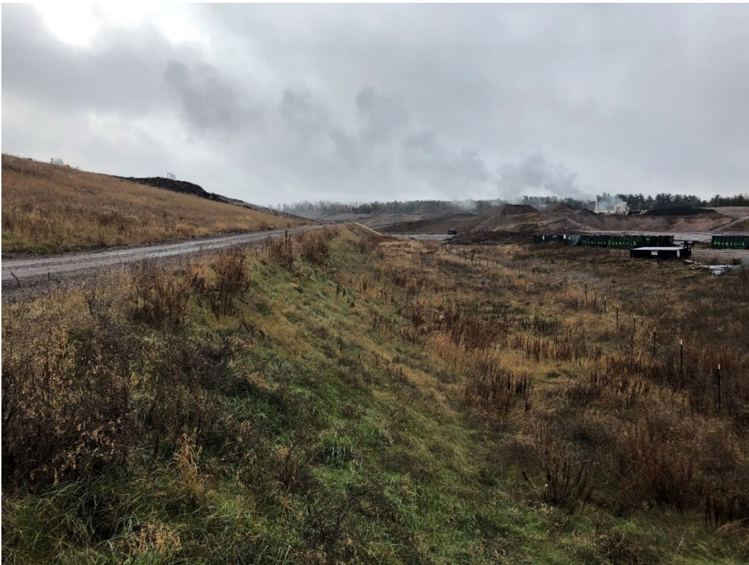
Photo 26: Location 10 – Looking South, Phase 2 Western Berm
