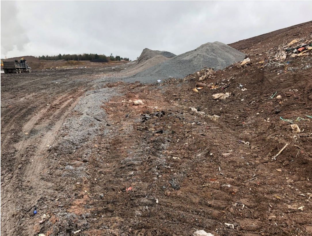
Photo 13: Location 7 – Looking West, Phase 4 Southern Waste Slope / 7A Interior Active Filling
