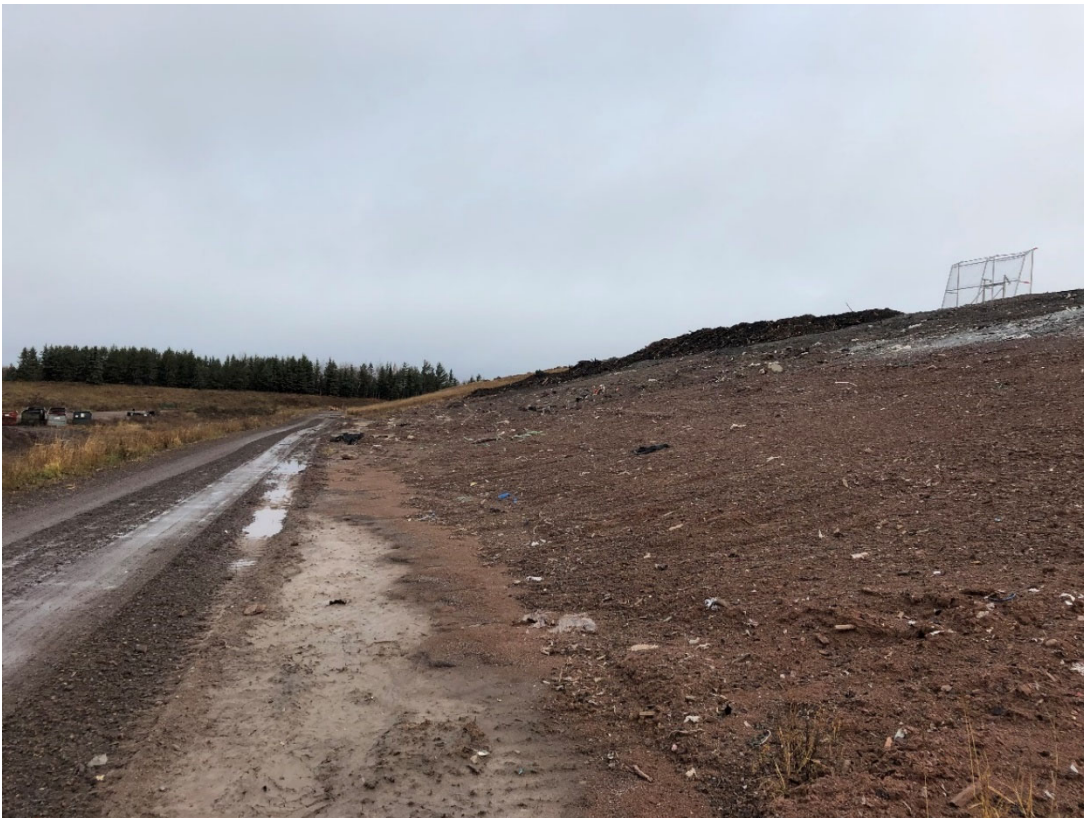
Photo 14: Location 8 – Looking North, Phase 3 Western Waste Slope
