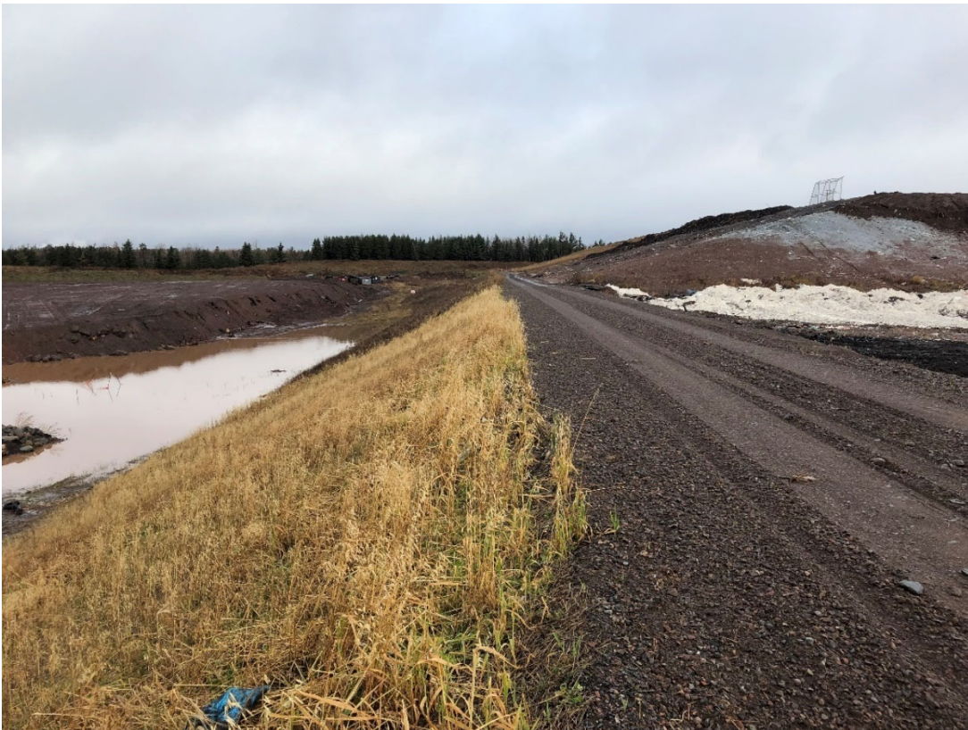
Photo 28: Location 11 – Looking North, Phase 6 Western LF Berm
