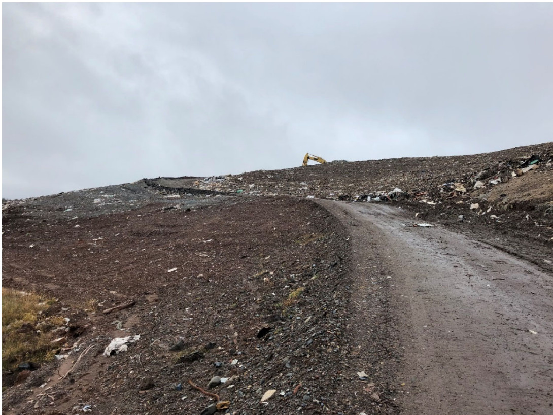
Photo 8: Location 5 – Looking Southwest, Phase 1 Southern Access Road
