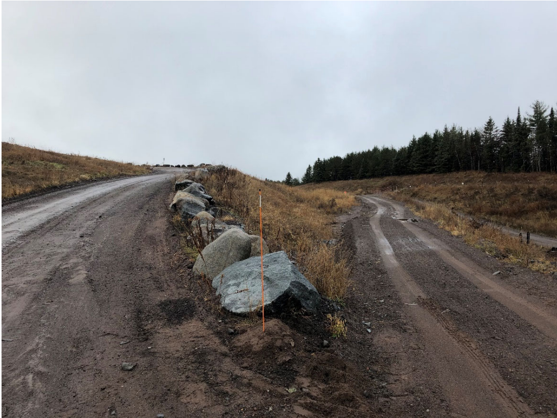
Photo 5: Location 3 – Looking West, Phase 2 Northern Waste Slope & Berm
