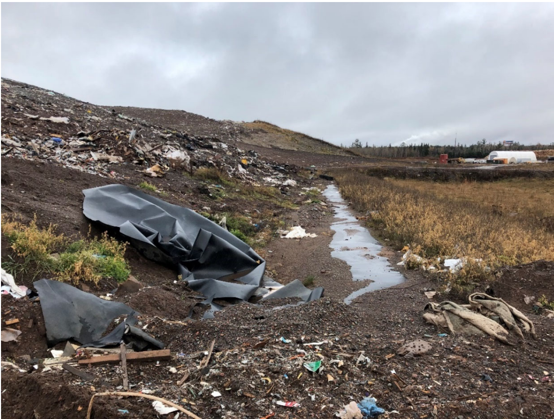
Photo 12: Location 7 – Looking North, Phase 4 Eastern LF Berm and Waste Slope
