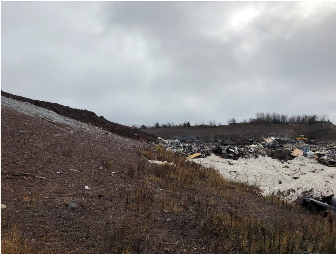
Photo 18: Location 8 – Looking East, Phase 3 Southern Interior Waste Slope
