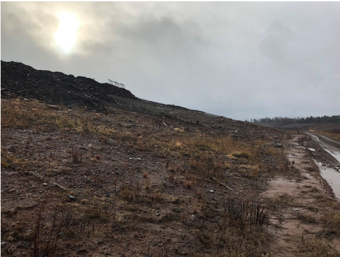
Photo 24: Location 9 – Looking South, Phase 3 Waste Slope
