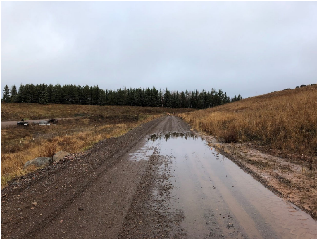
Photo 20: Location 9 – Looking North, Phase 2 Perimeter Road
