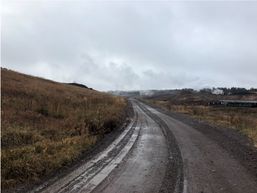
Photo 25: Location 10 – Looking South, Phase 2 Perimeter Road
