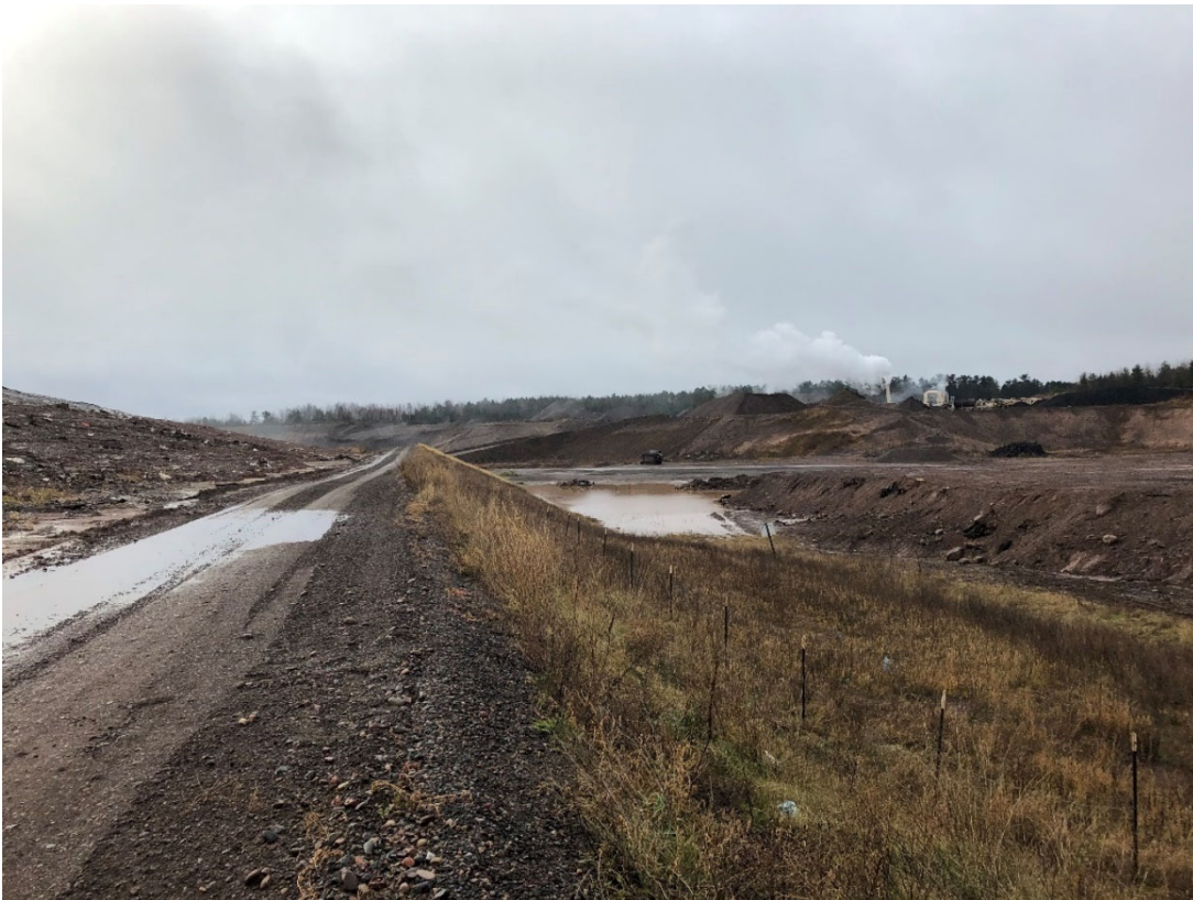
Photo 22: Location 9 – Looking South, Phase 3 Western Berm
