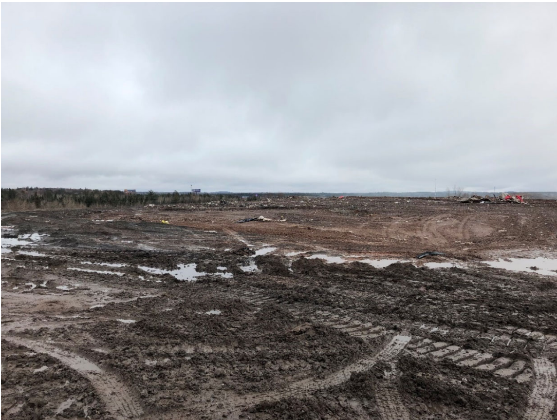
Photo 2: Location 1 – Looking Northeast, Phase 2/1 Upper Lifts
