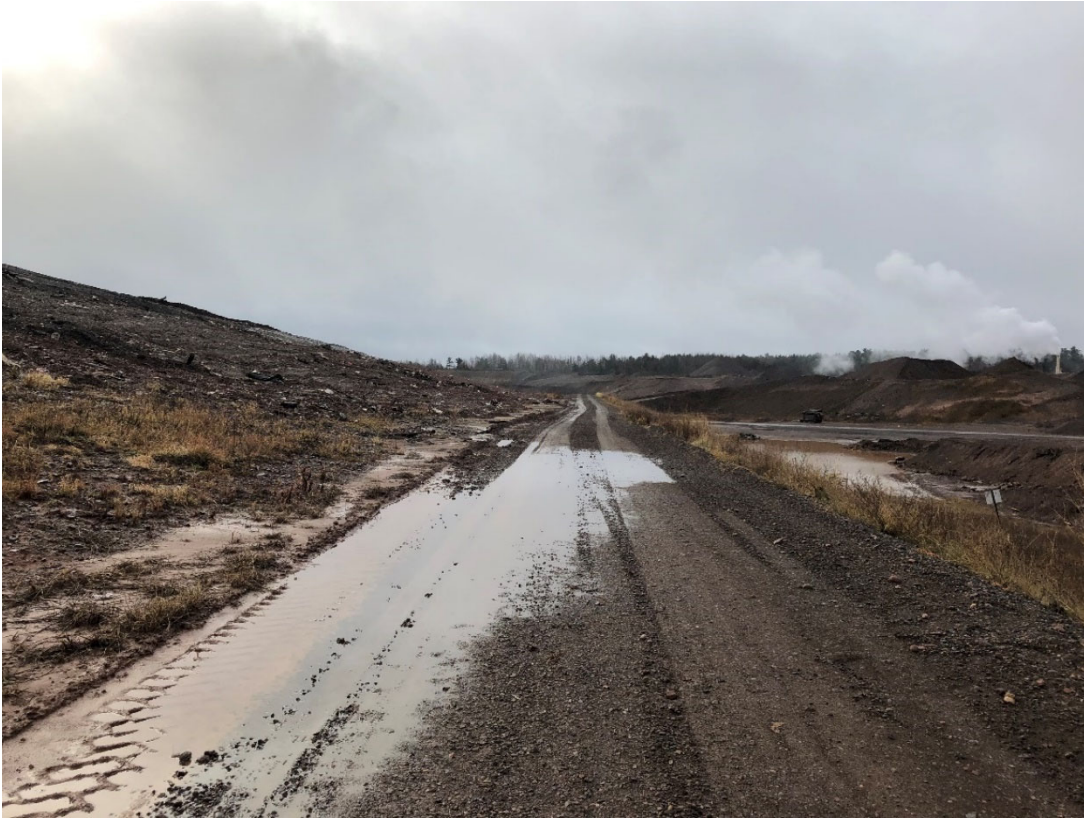
Photo 23: Location 9 – Looking South, Phase 3 Perimeter Road
