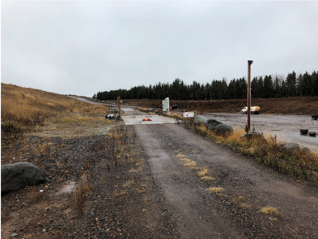
Photo 7: Location 4 – Looking West, Phase 1 Northern Berm
