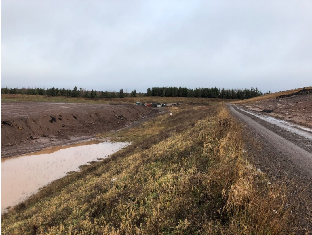
Photo 15: Location 8 – Looking North, Phase 3 LF Western Berm
