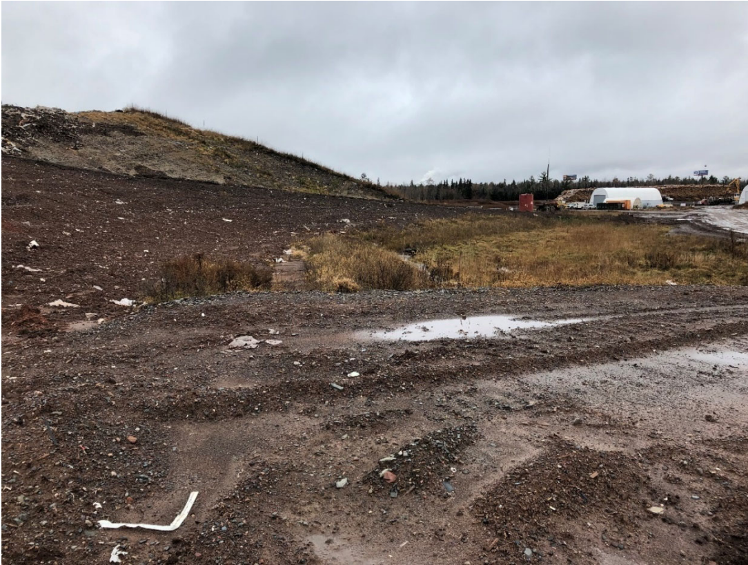
Photo 11: Location 6 – Looking North, Phase 4 Eastern Berm & Phase 1 Southeast Corner
