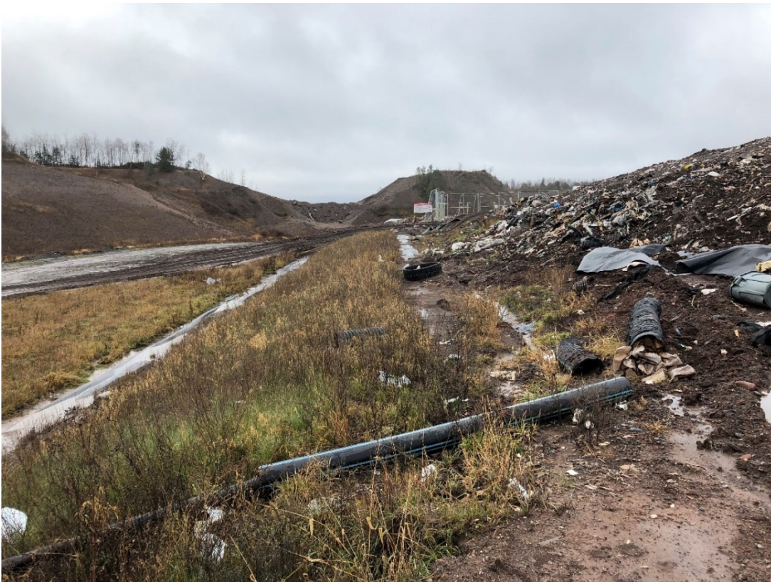
Photo 10: Location 6 – Looking South, Phase 4 Eastern Berm and Waste Slope
